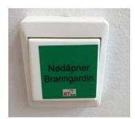
If you are stuck in the staircase between the 2nd and 3rd floor or 3rd and 4th floor, you can press the emergency opener for the fire curtain at the bottom of the stairs (see picture).
