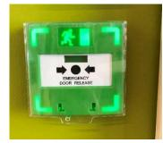
If the door to the escape route is locked - press the button for the emergency door release (see picture)
